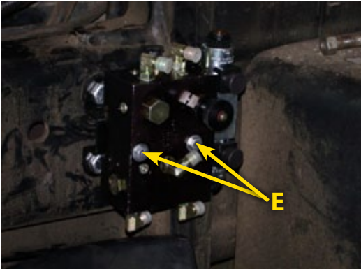
Figure 1-5: Installing the FieldPilot Valve
