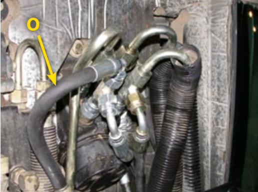
Figure 1-9: Replacing the Steel Pressure Line on Orbital
